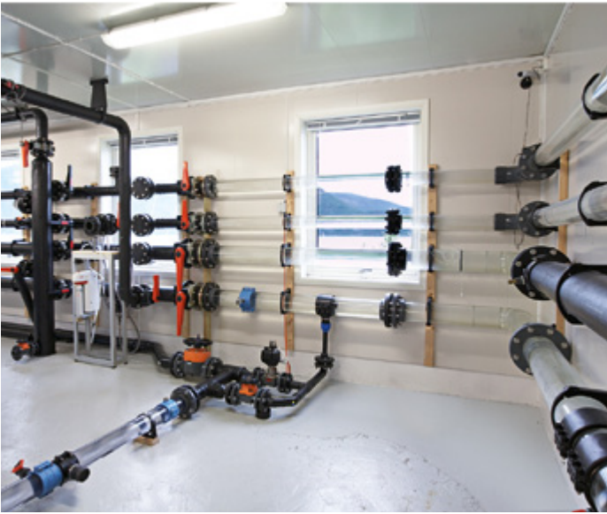
Transparent pipework to visualise optimum gas dissolution
