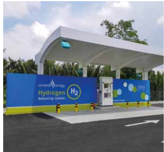
Refueling station in Sarawak (Malaysia)
